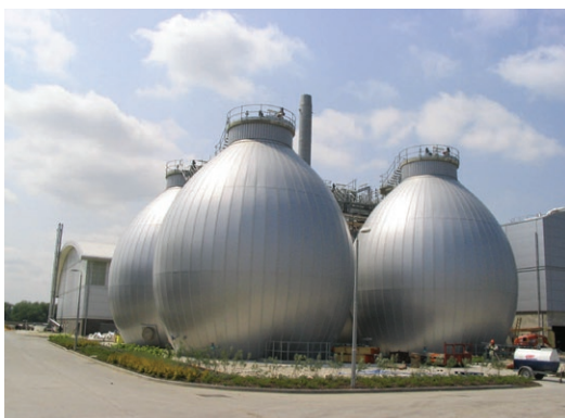
Reading, UK, sewage treatment works
