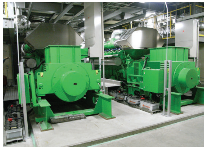
Yamagata, Japan, wood gas project 1 x JMS612, 1 x JMS 616
